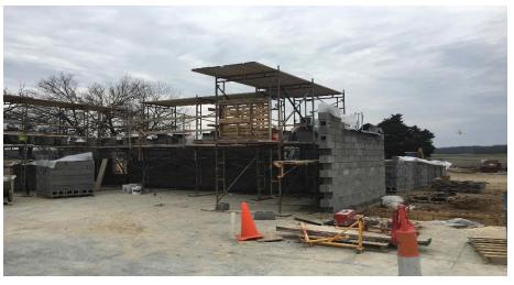
**Crosby Elementary:** Bearing walls in Area B continue to rise. The slab on grade at the Stage and Admin Area has been poured and the prep has begun for the Gym slab. The underground MEP in the kitchen has been completed.
