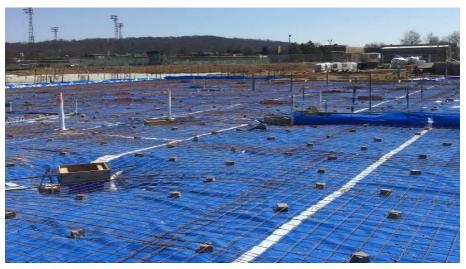
Miami Whitewater Campus: The South section of the Area B slab on grade has been prepped and will be poured this week. Foundation CMU and the underground MEP continues in Area A.
