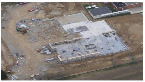
**Crosby Elementary:** Bearing walls in Area B continue to rise while the foundation CMU moves to the kitchen. At the end of the week, the slab on grade at the Gym will be poured and the underground plumbing will wrap up.
