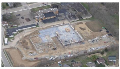
Harrison Elementary: Bearing walls in Area B continue to rise. The slab on grade prep at the Gym slab is finishing up to prepare for next weeks pour. The underground MEP in the kitchen continues. Bearing CMU continues in the kitchen and restroom core.
