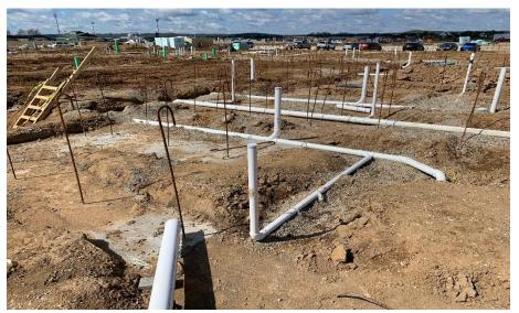
Harrison Junior High: Foundation block is being laid in Area A. The concrete footers in Area B are complete and work has begun in Area C. The underground plumbing in Area A has been finished and moved on to Area B while the primary electrical conduit is being installed across the site.
