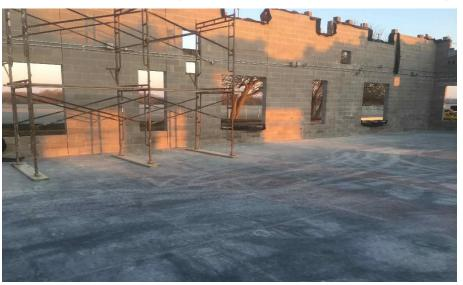
**Crosby Elementary:** Bearing walls in Area B continue to rise as the masons move to the mechanical and elevator core. The gym bearing walls in Area A have been laid out. Electrical rough-ins on exterior walls and the plumbing carriers continue to be installed across the building.
