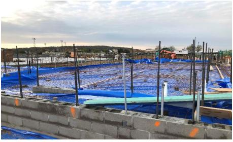
Miami Whitewater Campus: The masons have started the bearing walls in Area B. The slab on grade at the stage, admin, dining, and gym in Area A are being poured this week and the mechanical and kitchen area will be poured next week. Electrical and plumbing rough-ins have begun in Area B.
