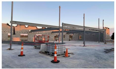
Crosby Elementary: Bearing walls in Area B continue to rise with the completion of the mechanical and elevator core. The masons will move to the bearing walls at the gym in Area A next week. Steel has been delivered and is being set in Area B to kick off Sequence #1!
