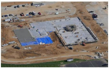
Miami Whitewater Campus: The bearing walls in Area B continue to rise. The final concrete slab on grade in the building has been poured in the mechanical and kitchen area. Electrical and plumbing rough-ins continues in Area B. Steel sequence #1 is slated to begin next week.
