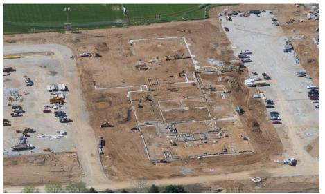
Harrison Junior High: The foundation block in Area A has been completed and will move to Area B while the concrete footers in Area C continue on. The underground plumbing in Area B has been installed and has shifted on to Area C. By the end of the week, the first concrete slab on grade will be poured for the Junior High!
