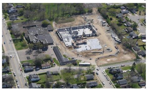
Harrison Elementary: The Area A stage and admin bearing walls continue to rise. Steel sequence #1 has been completed and sequence #2 is underway in Area B. Steel sequence #3 in Area A at the stage is being set simultaneously.
