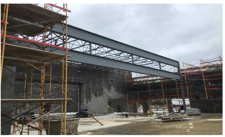
Harrison Elementary: The gym, mechanical, and kitchen bearing walls continue to rise in Area A. In Area B, half of the 2<sup>nd</sup> floor concrete slab will be poured this week. The 1<sup>st</sup> floor interior walls are being laid out to start framing next week. In-wall and above ceiling rough-in for MEP piping and duct continues in both Areas A and Area B.
