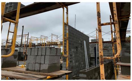
Harrison Junior High: Foundation block continues in Area C while bearing walls continue to rise in Area A. The concrete slab in the West half of Area B will be poured this week. MEP underground in Area C is near completion and MEP rough-ins are being installed in bearing block in Area A.
