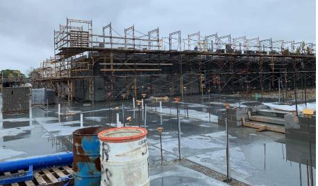
**Miami Whitewater Campus:** 1<sup>st</sup> floor bearing walls in Area B are nearing completion in preparation for 2<sup>nd</sup> floor steel. Steel columns and beams in the South half of Area B have been set and metal decking is being installed. Electrical and plumbing rough-ins are being installed in bearing block.
