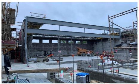
**Crosby Elementary:** The interior gym bearing walls and the cafeteria walls continue to rise in Area A. In the South half of Area B, steel has been set for the 2<sup>nd</sup> floor and metal decking is being installed. Electrical and plumbing roughins are being installed in bearing block.
