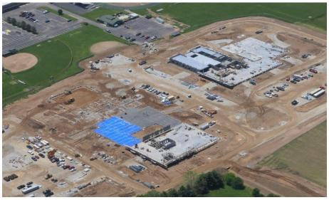
Harrison Junior High: Foundation block continues in Area C while bearing walls continue to rise in Area A. The concrete slab in the West half of Area B has been poured and the East half has been prepped for the next pour. MEP rough-ins are being installed in bearing block in Area A.
