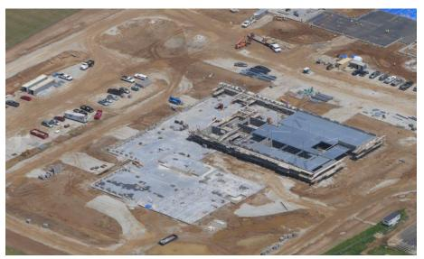
**Miami Whitewater Campus:** The North half of Area B bearing walls are nearing completion in preparation for 2<sup>nd</sup> floor steel. Steel in the South half of Area B is being detailed and metal decking is being installed. Electrical and plumbing rough-ins are being installed in bearing block.
