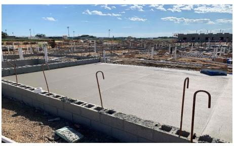
Harrison Junior High: In Area A, bearing walls continue to rise along with MEP rough-in for the academic wing, and structural steel sequence #1 has begun. In Area B, the East half of the concrete slab on grade was poured this week and slab prep has begun in Area C. Foundation block also continues in Area C.
