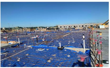
Harrison Junior High: In Area A, the 1<sup>st</sup> floor bearing walls and structural steel sequence #1 (East) have been completed in the academic wing. In-wall and above ceiling MEP rough-in continues. In Area C, the foundation block is complete and the gym, kitchen, and locker rooms are being prepped for next week's concrete pour.
