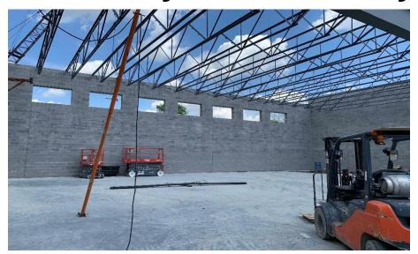
Crosby Elementary: In Area A, the stage bearing walls continue to rise and steel at the gym and mezzanine is being set. In Area B, the entire 2<sup>nd</sup> floor elevated concrete slab was poured and the 1<sup>st</sup> floor interior walls are being laid out. In-wall and above ceiling MEP rough-in continues in both Areas.
