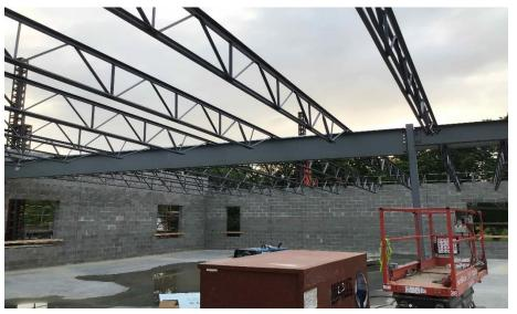
Harrison Elementary: In Area A, the elevated concrete slab at the 2<sup>nd</sup> floor mezzanine has been poured and the roof steel is being set. In Area B, the 2nd floor bearing walls are rising to the roof level and framing for the 1st floor interior walls continues. In-wall and above ceiling MEP rough-in continues in both Areas.
