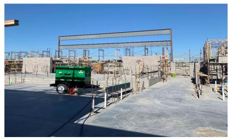
Miami Whitewater Elementary: The gym bearing walls are starting to rise after two steel beams were set in place at the gym entrance in Area A. In Area B, the North half of the 2nd floor steel is being set and the South half is prepped for this week's elevated concrete slab pour. In-wall and above ceiling MEP rough-in continues in both Areas.
