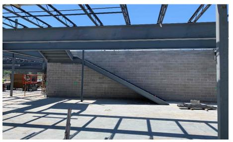
Miami Whitewater Elementary: The gym bearing walls continue to rise in Area A. In Area B, metal stairs have been installed up to the 2<sup>nd</sup> floor and layout has begun for the 1<sup>st</sup> floor interior walls. The North half of the 2nd floor steel is being set. In-wall and above ceiling MEP rough-in continues in both Areas.
