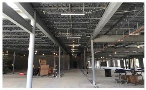
Crosby Elementary: In Area A, the stage bearing walls continue to rise and the mezzanine concrete floor has been poured. The steel joists in the gym are being detailed in preparation for roof decking. In Area B, the 1st floor interior walls and door frames are being framed and set. In-wall and above ceiling MEP rough-in continues in both Areas.
