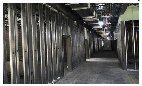
Harrison Elementary: The indoor air-handling units have been delivered and set into place. In Area B, the 2nd floor bearing walls have reached the roof level and the roof steel has been set. The interior wall framing at the 1<sup>st</sup> floor is nearly complete and the 2<sup>nd</sup> floor is starting layout. In-wall and above ceiling MEP rough-in continues in both Areas.
