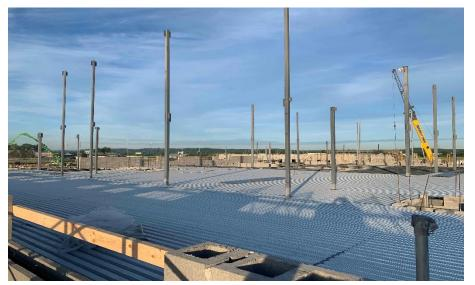
Harrison Junior High: Structural steel is being set in the West half of the academic wing and bearing block walls are rising in Area B. In Area C, the gym, kitchen, and locker room concrete floors were poured and the admin area is being prepped for next week's concrete pour. In-wall and above ceiling MEP rough-in continues.
