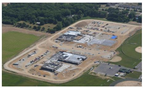
Miami Whitewater Elementary: The gym bearing walls continue to rise in Area A. In Area B, the 1<sup>st</sup> floor interior walls are being framed in and door frames are being set. Metal decking in the North half of the 2nd floor is being installed and prepped for the upcoming elevated concrete pour. In-wall and above ceiling MEP rough-in continues in both Areas.
