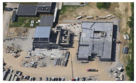
Crosby Elementary: In Area A, the stage bearing walls continue to rise and the mechanical concrete pad at the mezzanine has been poured. In Area B, the 2<sup>nd</sup> floor block walls are rising to the roof level and the elevator shaft has been built. The 1<sup>st</sup> floor interior walls and door frames are being framed and set. In-wall and above ceiling MEP rough-in continues in both Areas.
