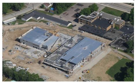
Harrison Elementary: The Area A kitchen and mechanical block walls are being laid. In Area B, the 2nd floor roof decking is being installed and metal stairs are being set. The interior wall framing is complete at the 1st floor and the 2nd floor framing has begun. In-wall and above ceiling MEP rough-in continues in both Areas.
