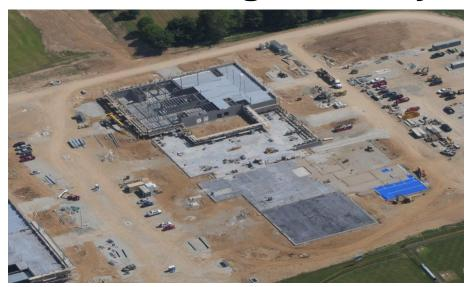
Harrison Junior High: 2<sup>nd</sup> floor metal decking is being installed in the West half of the academic wing and bearing block walls continue to rise in Area B. In Area C, the admin concrete floor has been poured and bearing block is being laid out in the kitchen and gym. In-wall and above ceiling MEP rough-in continues.
