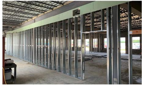
Miami Whitewater Elementary: The gym and stage bearing walls continue to rise and the roof steel has been set at the gym in Area A. In Area B, the 1st floor interior walls have been framed in and the door frames are being set. The elevated concrete slab in the North half of the 2nd floor and the air handling unit concrete pads have been poured. In-wall and above ceiling MEP rough-in continues.
