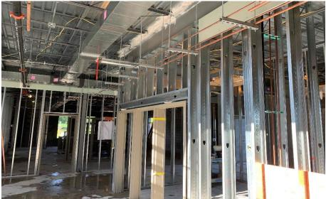
**Crosby Elementary:** In Area A, the roofing material has been delivered and the metal roof decking is being installed in the gym, cafeteria, and stage. The main entrance bearing block walls are being laid. In Area B, the 2<sup>nd</sup> floor block walls are complete up to the roof level. HVAC duct and sprinkler lines have been installed in Area B level 1. In-wall and above ceiling MEP rough-in continues in both Areas.
