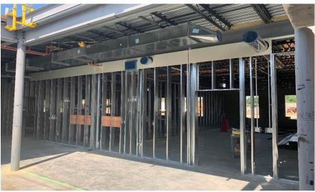
Miami Whitewater Elementary: The stage bearing block walls continue to rise and the roof steel has been set at the gym in Area A. The air handling units were delivered this week and installation has begun. Inwall and above ceiling MEP rough-in continues throughout Area B.
