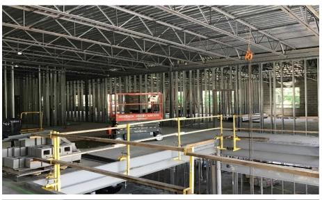
Harrison Elementary: The bearing block walls in the Area A administration wing continue to rise. In Area B, the roof will be completed and the window openings will be covered this week. Metal stair installation continues in the stairwells. The 2<sup>nd</sup> floor interior walls and door frames are being framed and set. In-wall and above ceiling MEP rough-in continues in both Areas.
