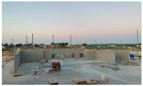
Harrison Junior High: In the academic wing, the 2<sup>nd</sup> floor bearing walls are rising while the 1<sup>st</sup> floor interior walls are being framed in. The structural steel in the West half of Area B is being set as the East half prepares for an elevated concrete pour. Precast concrete planks have been placed for the 2<sup>nd</sup> floor Area C gym. In-wall and above ceiling MEP rough-in continues.
