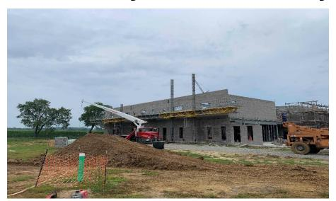
Crosby Elementary: In Area A, the roof is being installed at the gym and cafeteria while bearing block and brick is being laid at the main entrance, kitchen, and mechanical room. In Area B, roof steel is being set above the academic wing. In-wall and above ceiling MEP rough-in continues in both Areas.
