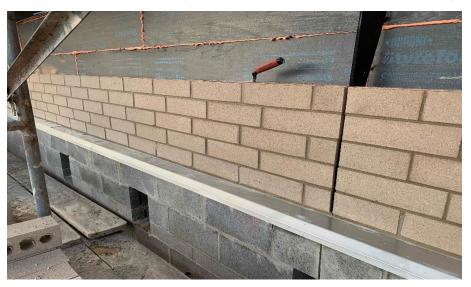
**Crosby Elementary:** In Area A, bearing block walls are being laid in the mechanical room and administration area while brick is being laid over the kitchen and mechanical room roof. In Area B, roof steel and decking is being set above the academic wing. In-wall and above ceiling MEP roughin continues in both Areas.
