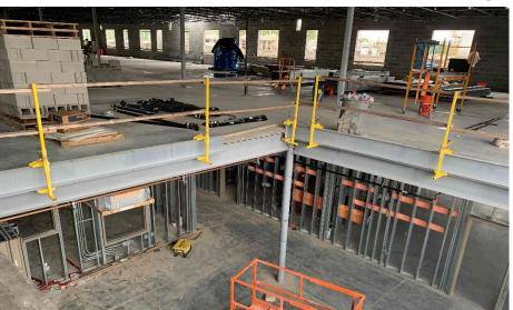
Miami Whitewater Elementary: Bearing block walls are being laid in the kitchen, mechanical room, and administration area in Area A. In Area B, structural steel roof decking is complete as roof installation continues. The interior walls on the 2<sup>nd</sup> floor are being laid out. In-wall and above ceiling MEP rough-in continues throughout Area B.
