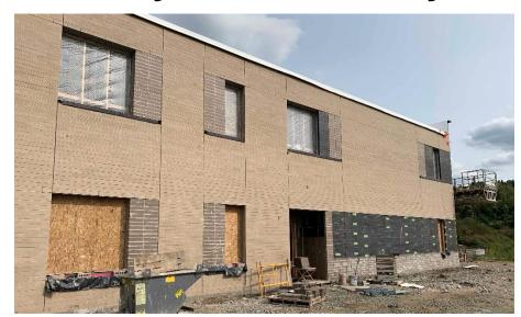
Crosby Elementary: In Area B, drywall is being hung on the 1st floor and interior CMU block walls are being laid around the restrooms on the 2nd floor. In Area A, the kitchen roof is being installed and steel is being erected in the administration area. Brick is being laid on the North and East wall of Area B. In-wall and above ceiling MEP rough-in continues in both Areas.
