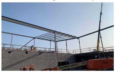
Harrison Junior High: Interior walls on level 2 of Area A and level 1 of Area B are being laid out and framed. Bearing block walls continue to rise in all three Areas while roof steel is being set on the 2<sup>nd</sup> floor of Area B. The concrete seating for outdoor classes has been poured in the courtyard. In-wall and above ceiling MEP rough-in continues in all Areas.
