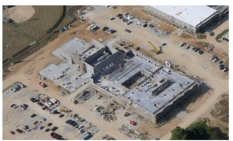
Harrison Junior High: Bearing block walls continue to rise in Areas A and C while roof steel is being set on the 2<sup>nd</sup> floor of Area B. Concrete work has shifted from the courtyard to the bus lot sidewalks. In-wall and above ceiling MEP rough-in continues in all Areas and the last DOAS unit has been set in the building.
