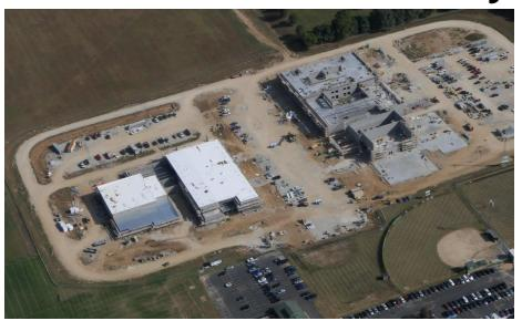
Miami Whitewater Elementary: Metal roof decking has been installed and detailed in the kitchen, mechanical room, administration, and art room. In Area B, the interior walls on the 2<sup>nd</sup> floor have been framed as the 1<sup>st</sup> floor preps for drywall next week. Brick continues on the East wall of Area B. Above ceiling MEP rough-in continues in both Areas.
