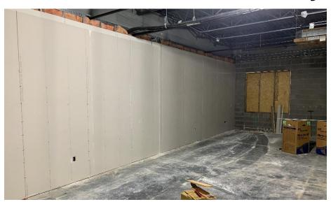
Miami Whitewater Elementary: The roof is being installed above the kitchen, mechanical room, administration, and art room in Area A. The interior walls are being laid out and framed in Area A and drywall is being hung on the 1st floor of Area B. Brick continues on the East wall of Area B. Above ceiling and in-wall MEP rough-in continues in both Areas.
