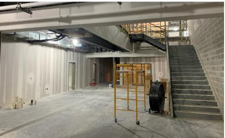
**Miami Whitewater Elementary:** The interior kitchen and mechanical room block walls are being built in Area A. In Area B, the 1<sup>st</sup> floor drywall walls are being finished as the drywall on the 2<sup>nd</sup> floor is being hung. Above ceiling and in-wall MEP rough-in continues in both Areas. The base coat of asphalt is complete at the Miami Whitewater & Junior High Campus.
