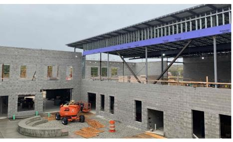
Harrison Junior High: Roof steel is being set on the West half of Area A as the East half bearing block walls are nearly complete. Roof installation begins above Area B and the exterior courtyard soffits are being framed in. The main gym walls are beginning to rise in Area C and In-wall and above ceiling MEP rough-in continues. The base coat of asphalt is complete at the Miami Whitewater & Junior High Campus.
