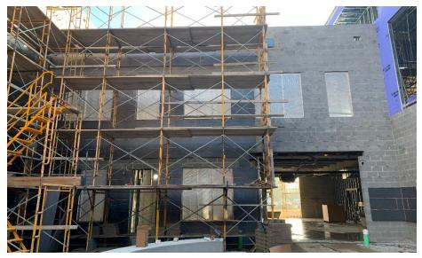
Harrison Junior High: Roof steel erection is complete above the auxiliary gym while roof installation continues over Areas A & B. Block walls are complete at the main gym and continue to rise in the administration wing. The interior drywall walls are being framed on the 3<sup>rd</sup> floor of Area A and 2<sup>nd</sup> floor of Area B. In-wall and above ceiling MEP rough-in continues in all Areas. Brick work has begun in the courtyard!
