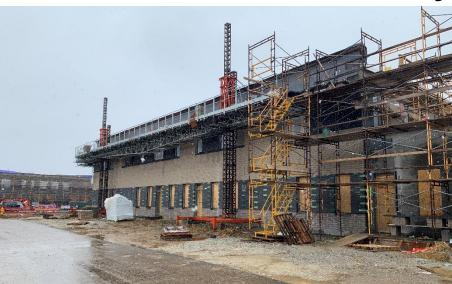
**Miami Whitewater Elementary:** Drywall finishing in the administration wing has been completed and the walls are being primed and painted. In Area B, classroom cabinets are being installed on the 1<sup>st</sup> floor while ceiling grid installation is complete on the 2<sup>nd</sup> floor. Brick continues along the Area B walls while the South entrance canopy steel has been erected. Overhead MEP rough-in continues.
