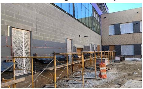
Harrison Junior High: Roof steel is complete above the administration wing while roofing continues above Areas B & C. Brick continues in the courtyard and on the West wall of Areas A & B. Drywall is being hung on the 1<sup>st</sup> floor of Area A while drywall finishing is complete on the 2<sup>nd</sup> floor. In-wall and above ceiling MEP rough-in continues in all Areas.
