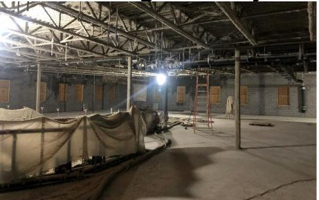
Harrison Junior High: Roof installation continues above the administration area while the fireproofing underneath is nearly completed. Brick continues along the North wall of Area A. Drywall is being hung on the 2<sup>nd</sup> floor of Area B and being finished on the 3<sup>rd</sup> floor of Area A. Painting, lighting, and ceiling grid installation continues on the 1<sup>st</sup> and 2<sup>nd</sup> floors of Area A.
