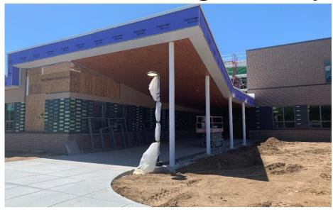
Harrison Junior High: Soft flooring installation continues in Area B and Admin while the auxiliary gym flooring is laid. The main entrance storefronts and music room curtain walls are being installed. Final painting continues throughout the building. Elevator installation is ongoing. Asphalt striping continues in the parking lot. The first wave of furniture was delivered this week!
